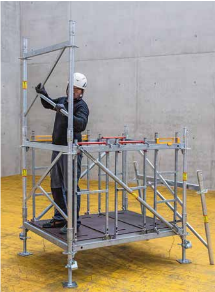
The frame slides into the end position under its own weight.
