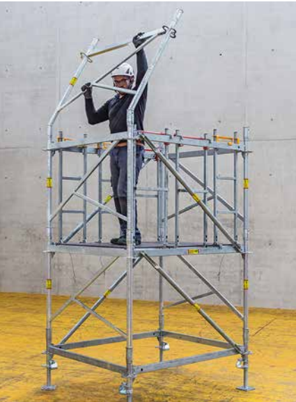
After attaching the frame to the tulip under 45°, the frame is turned into a vertical position.
