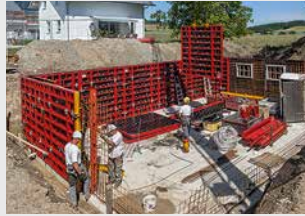
Wall Formwork
