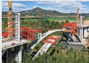
Bridge Formwork
