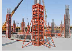
Column Formwork
