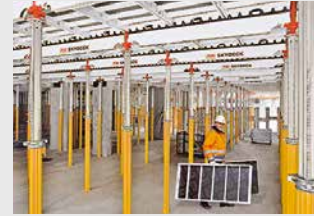
Slab Formwork
