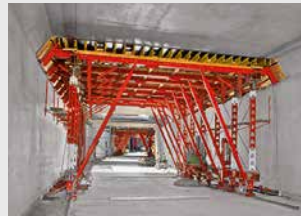
Tunnel Formwork
