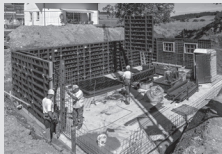
Wall Formwork
