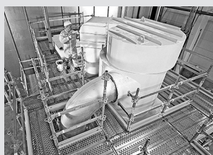
Working scaffolds industry
