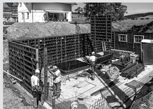
Wall formwork
