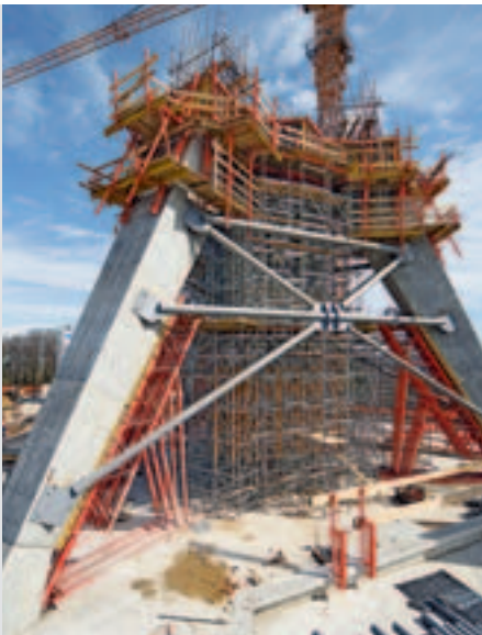
Same system components for providing temporary support for the structure as well as for climbing scaffold application.
