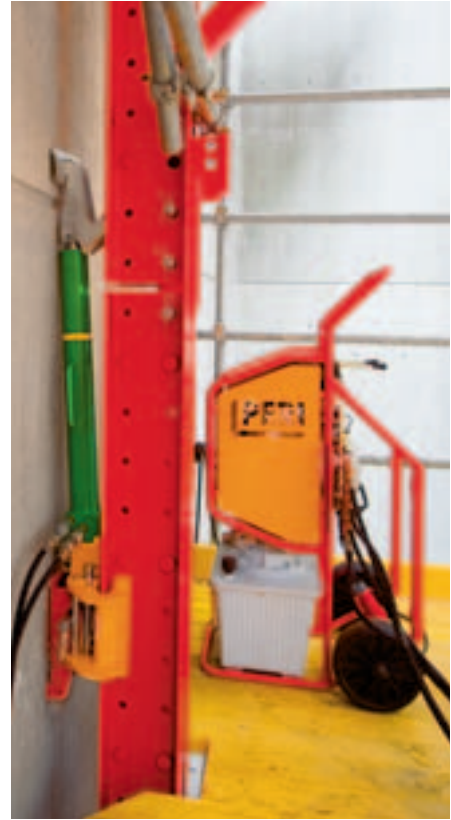
RCS climbing rail with hydraulic climbing device.
