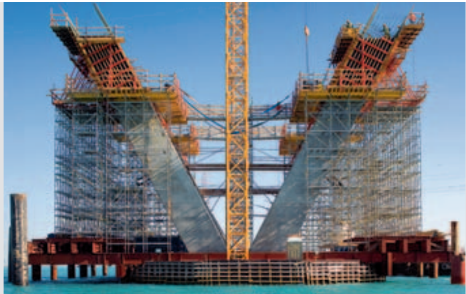
Adaptable trusses for transferring fresh concrete loads and as temporary structure support.
