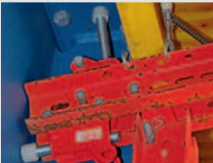
Support spindles for optimal adjustment to the bridge cross-section with an adjustment range of +/- 10 cm.
