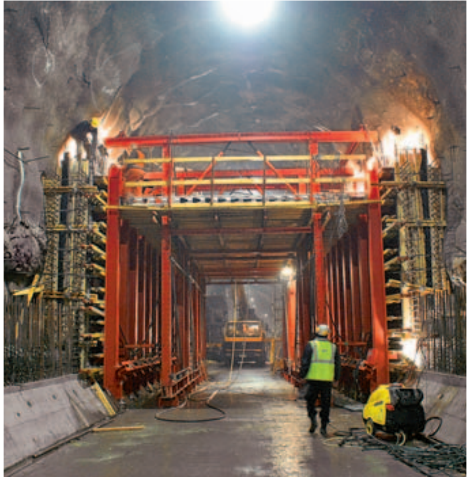
The first section with the bottom slab and starter has already been concreted.
