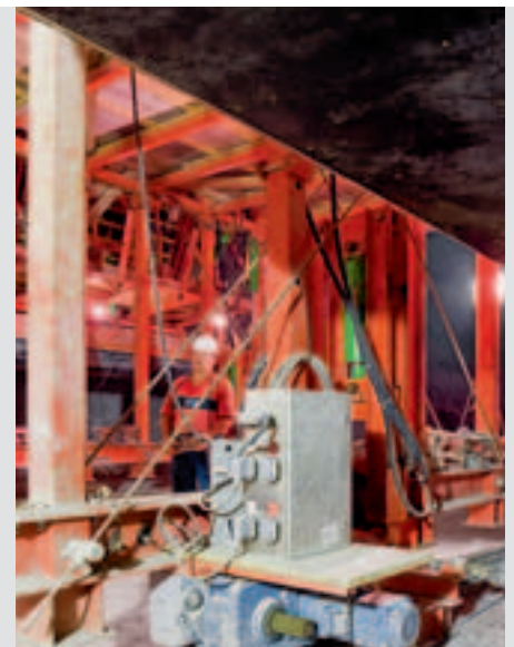
Optional VARIOKIT accessories such as hydraulic winches, electric drive units, lifting and lowering units and hydraulic cylinders for operating the wall and slab formwork elements are available in the VARIOKIT construction kit and, if necessary, are planned according to project requirements.
