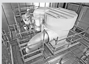
Working scaffolds industry
