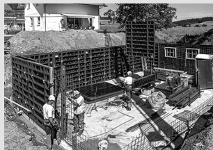
Wall formwork
