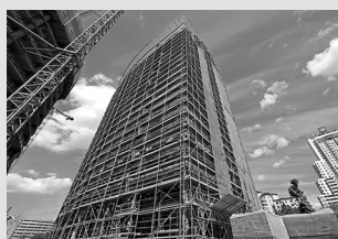
Working scaffolds facade
