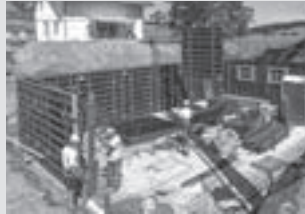
Wall Formwork
