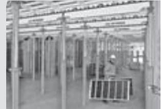
Slab Formwork
