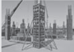
Column Formwork
