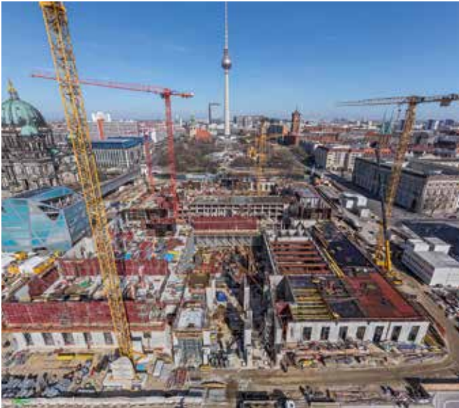
More than 6,000 m 2 of MAXIMO Panel Formwork materials were in simultaneous use during construction of Berlin's City Palace.
