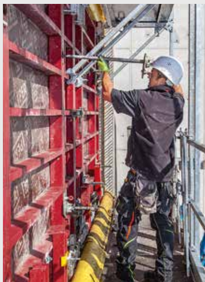
All anchors are easily accessible, while the yellow rubber lip protects the element against dirt.
