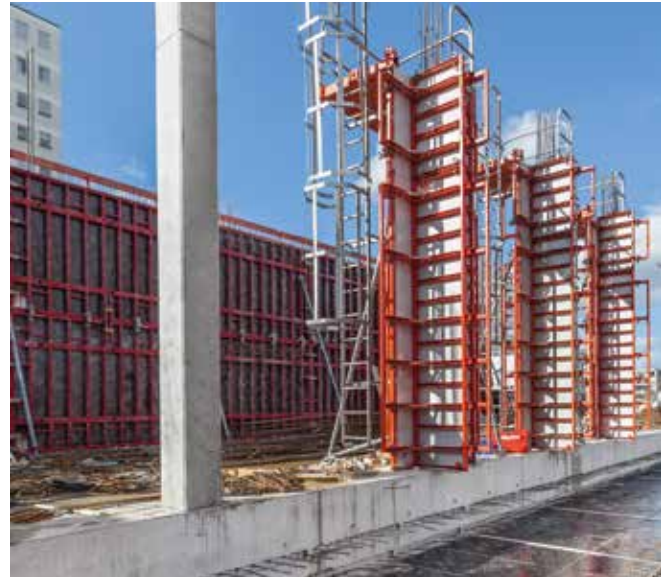
The walls of the "am Hirschgarten" urban district were formed in no time at all using MAXIMO Panel Formwork.
