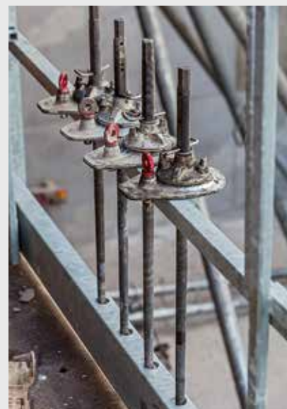
You can suspend the anchors directly on the guardrails. Once the unit has been moved, they are ready for installation again.
