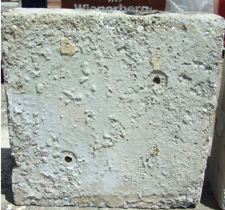
Photo 7 Exposed face after fire test
