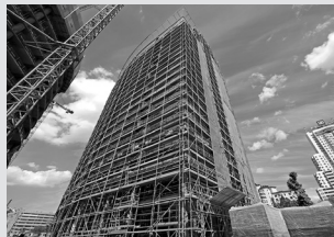
Working scaffolds facade
