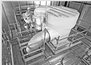
Working scaffolds industry
