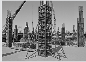
Column formwork
