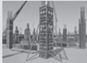
Column Formwork
