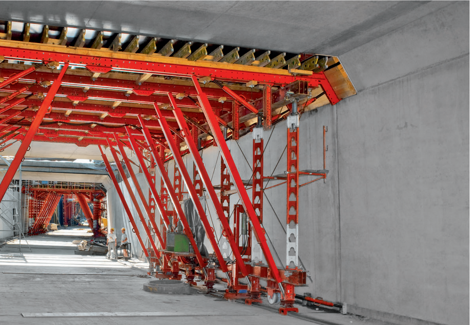
Clearly visible are the 2 separate concreting cycles, the wall on the left and the slab on the right. Both sets of formwork are designed as mobile units.
