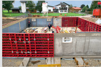
Wall Formwork
