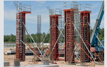
Column Formwork
