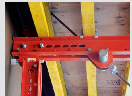
Tie Yoke Head SRU with DW 15 tie rod, can be operated from the underside of the bridge.
