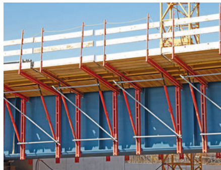
The bracket units with side protection mounted on the steel girders serve, at the same time, as guardrails.
