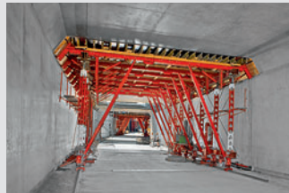
Tunnel Formwork
