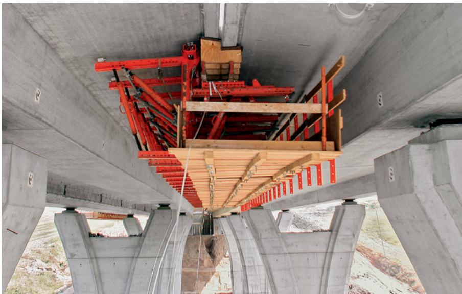
Optimal and flexible adjustment to the bridge geometry for the construction of the middle parapet.
