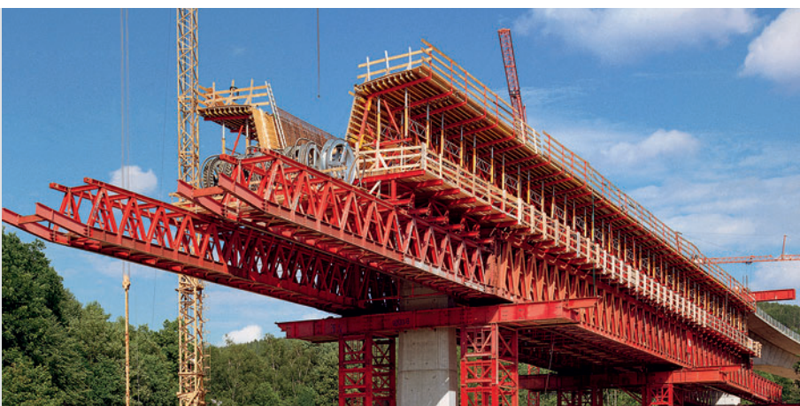
The underslung launched traveller can also be supplemented with system formwork thus ensuring cost-effective use. For moving, the traveller and formwork are firstly pushed sideways, then moved forward in a longitudinal direction and subsequently realigned.
