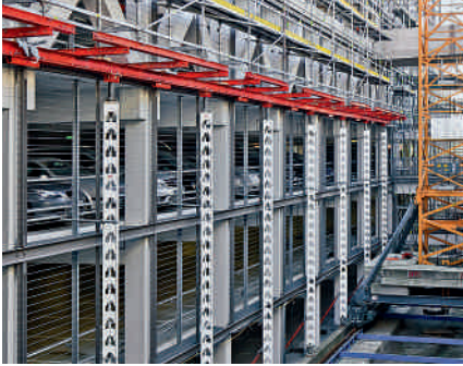
HD 200 Heavy-Duty Props as a space-saving solution: 8 m high props transfer the loads from a working and safety scaffold in a confined area.
