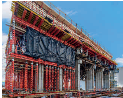
HD 200 Heavy-Duty Props as a full-surface shoring structure. The HD 200 sections were joined together, also at great heights, in order to safely transfer the loads of the 3.20 m thick reinforced concrete slab for the generator.
