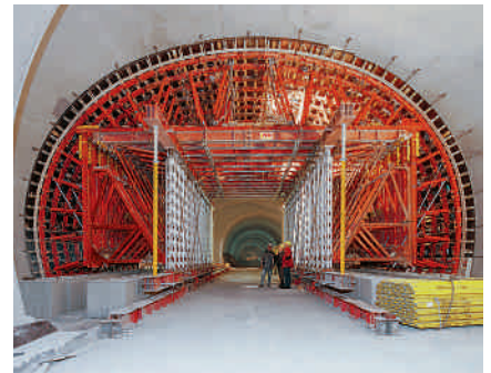
The moveable longitudinal truss – taken from the HD 200 heavy-duty system – for this tunnel was designed as a portal. This allowed a continuous flow of site traffic at all times.
