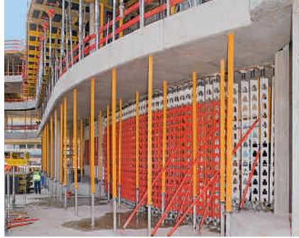
A lightweight but load-bearing solution: Below the shear walls, HD 200 Heavy-Duty Props transfer linear loads of up to 400 kN/m into the bottom plate.
