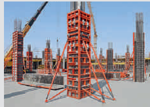
Column Formwork
