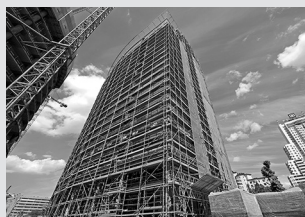
Working scaffolds for facades
