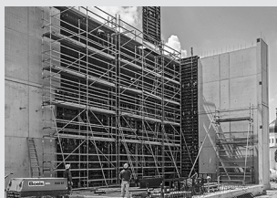
Working scaffolds for construction
