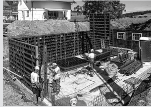
Wall formwork
