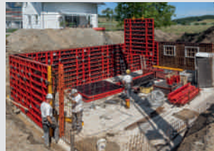
Wall Formwork
