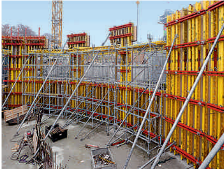
Use with VARIO GT 24 Girder Wall Formwork The Arctic Ring, Copenhagen Zoo, Denmark.
