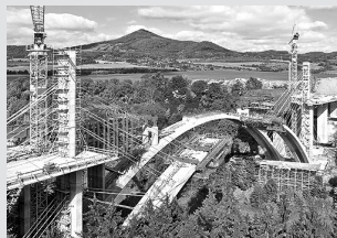
Bridge formwork
