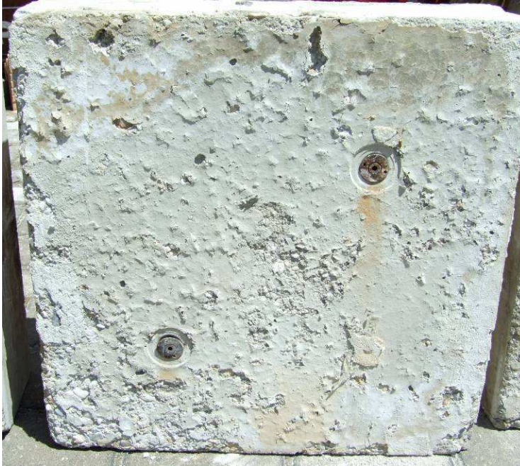
Photo 7 Exposed face after fire test
