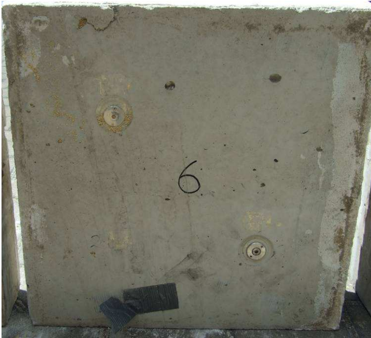
Photo 5 Unexposed face after fire test
