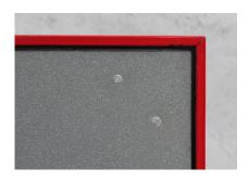
The nailed formlining leaves an inconspicuous negative imprint in the concrete finish.
