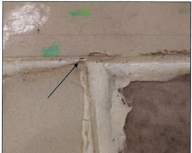
Image 7: spot of water permeability
