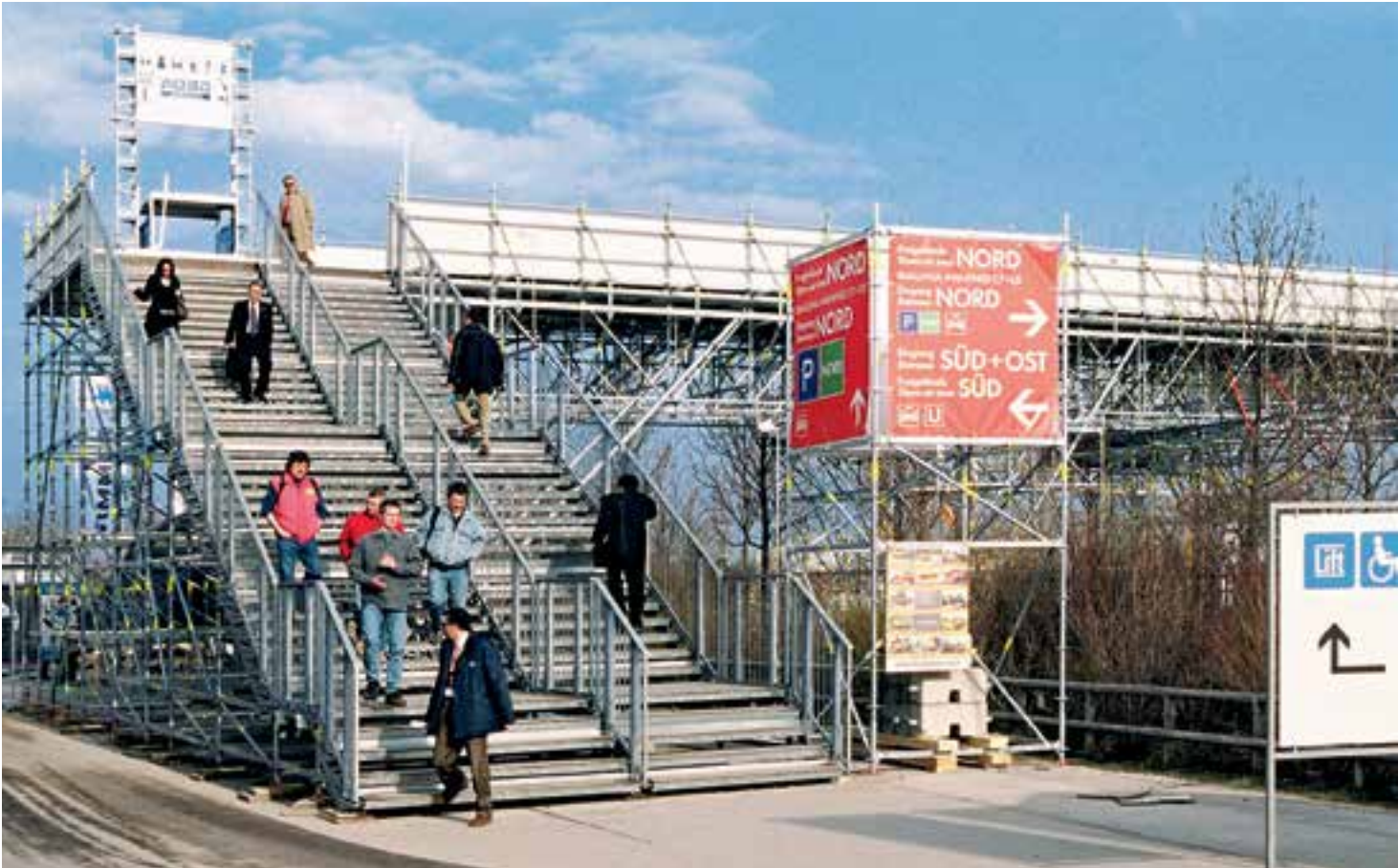
Solution for a trade fair: stairway leading to a pedestrian bridge over a multi-lane road with separate routes for up and down.
