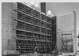
Working scaffolds construction
