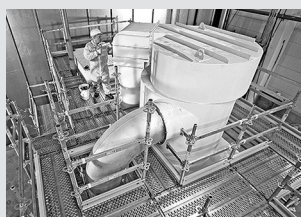
Working scaffolds industry
