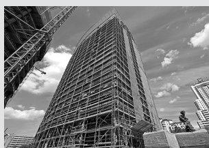
Working scaffolds facade
