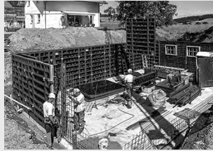
Wall Formwork
