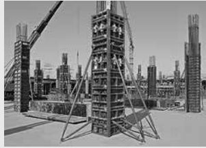
Column formwork
