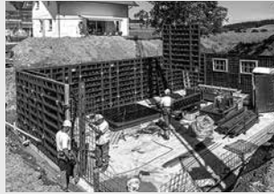
Wall formwork
