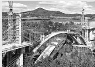
Bridge formwork
