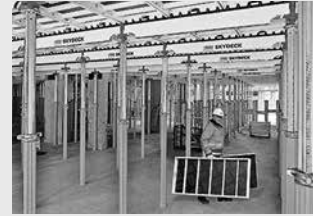
Slab formwork
