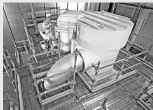
Working scaffolds industry
