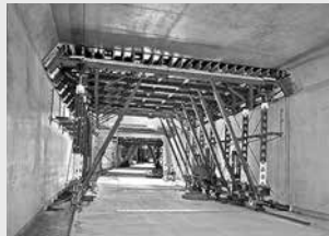
Tunnel formwork
