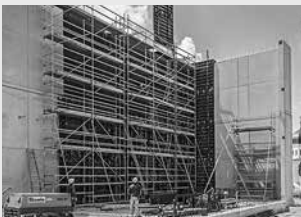
Working scaffolds construction
