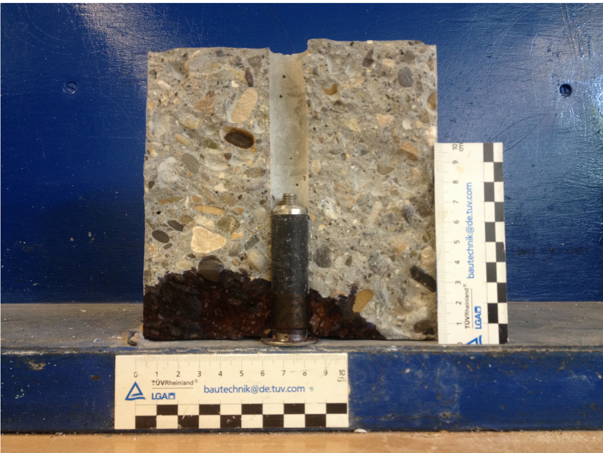
Fig. No. 9 Sample S6 Water penetration
