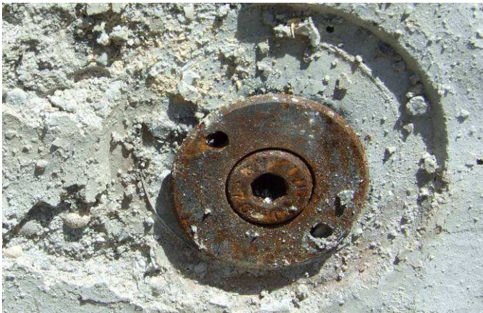
Photo 8 Screw plug "Schraubstopfen MX 15-50 MF-LS" Exposed face after fire test
