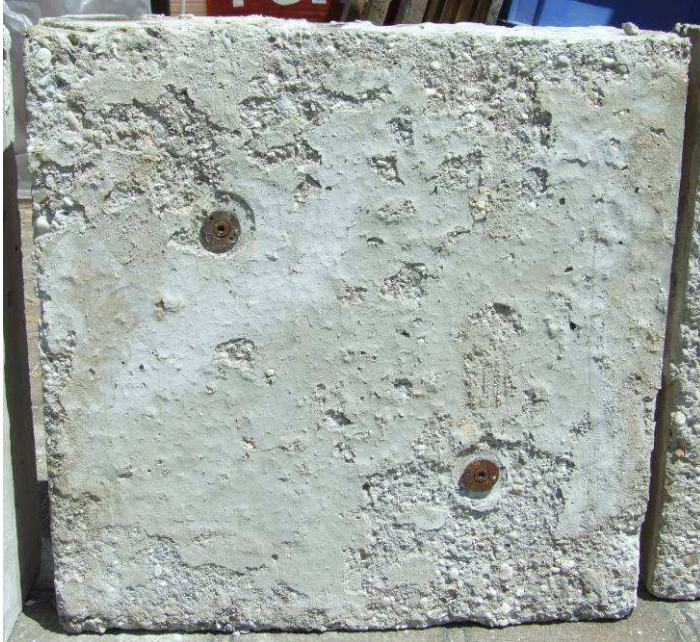
Photo 7 Exposed face after fire test
