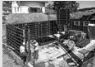
Wall Formwork
