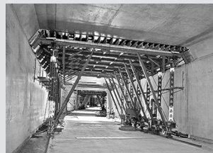
Tunnel Formwork
