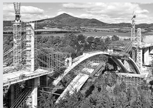
Bridge Formwork
