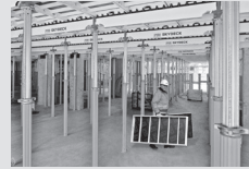
Slab Formwork
