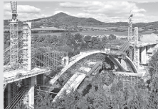
Bridge Formwork
