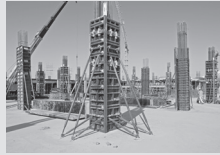
Column Formwork
