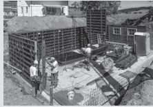
Wall Formwork
