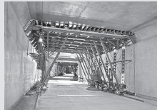
Tunnel Formwork
