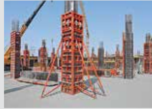
Column Formwork
