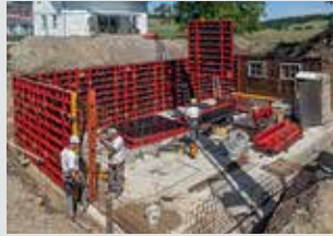
Wall Formwork
