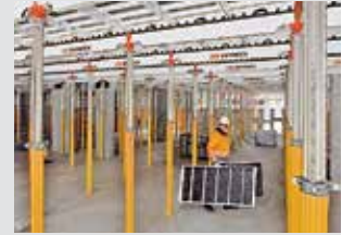
Slab Formwork
