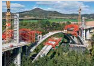
Bridge Formwork
