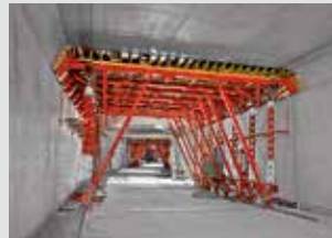
Tunnel Formwork
