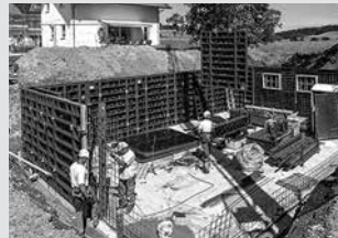
Wall Formwork
