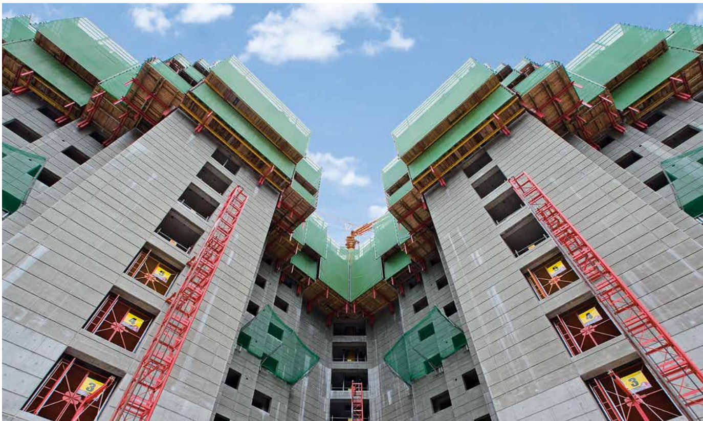
Complicated layouts can also be cost-effectively climbed with the RCS C formwork scaffold thanks to the flexibility – rail-guided and crane-independently.
