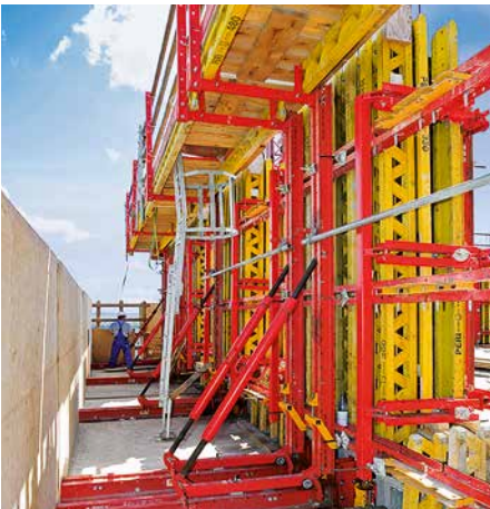
This column formwork in the facade area climbs crane-independently upwards with the RCS Self-Climbing Technology. At the same time, the enclosure provides protection against wind and weather.
