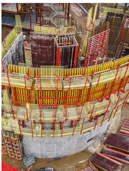
The use of the lightweight rail-guided climbing formwork for a circular structure with the VARIO GT 24 Girder Wall Formwork.
