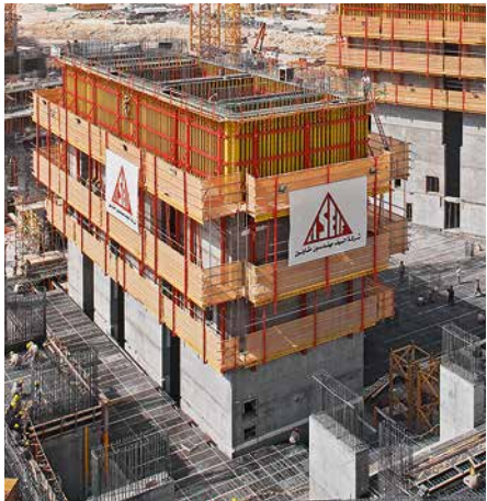
Safe working conditions with continuous lateral and rear protection on and under the RCS C Climbing Formwork.
