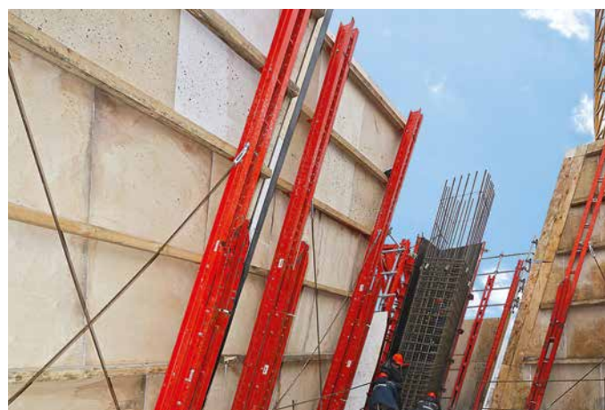
Here, the climbing rails of RCS Protection Panel follow the inclined form of the structure. Special slab shoes guarantee secure connection of the rails to the structure.
